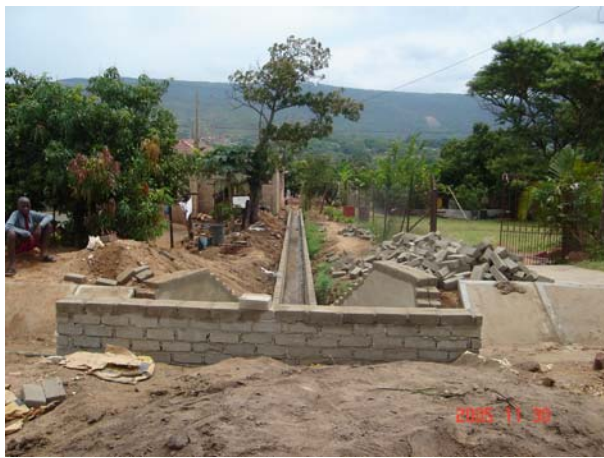
Refurbishment of street at Highpoint in Ga-Kgapane
